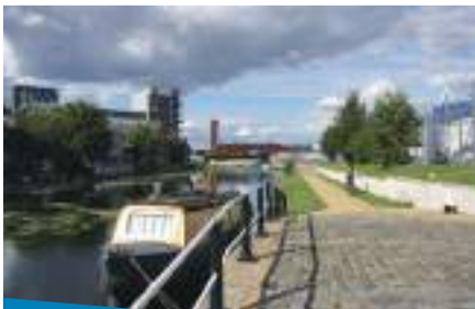
River Lee Navigation lifting point
