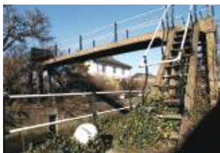
City Mill Lock
