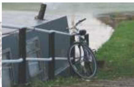
1.f Lifting point on River Lee Navigation
