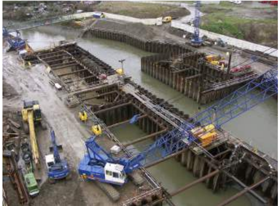
Construction of Three Mills Lock
