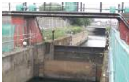
Carpenters Road Lock
