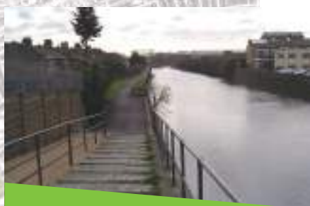
2.e Steps on Three Mills Wall River
