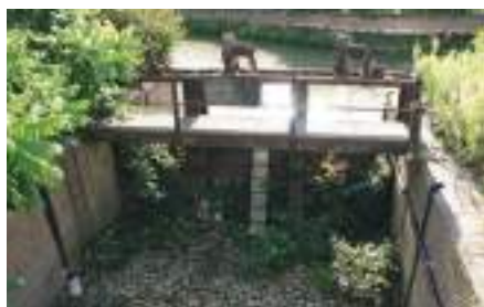
City Mill Sluice
