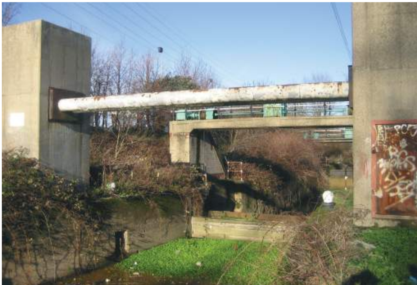
Carpenters Road Lock
